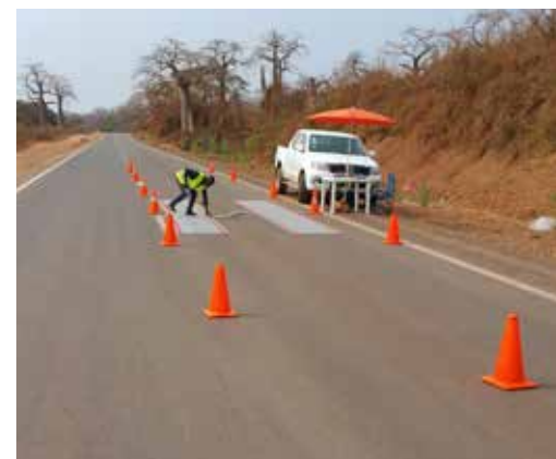
Pre-selection with low speed WIM system in Angola
